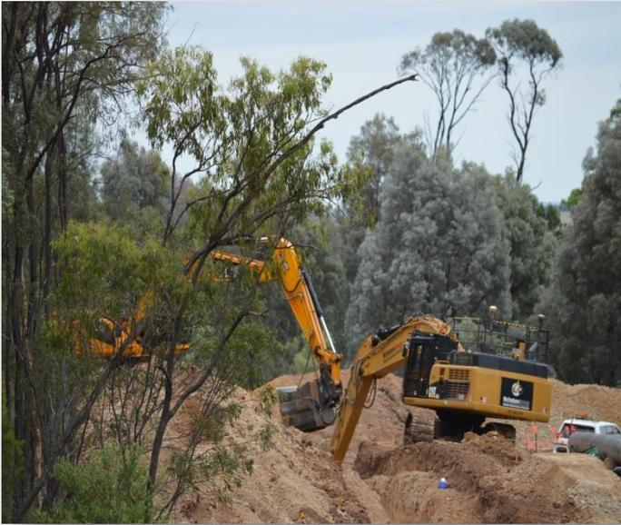
There was also a large number of roads, water courses and existing pipelines to be crossed, 155 in total, many of these were existing live pipelines and work was carried out under strict permit conditions and without incident. The numerous watercourses were constructed using open cut methodology but were subject to the strict licensing conditions of the Queensland Government.
